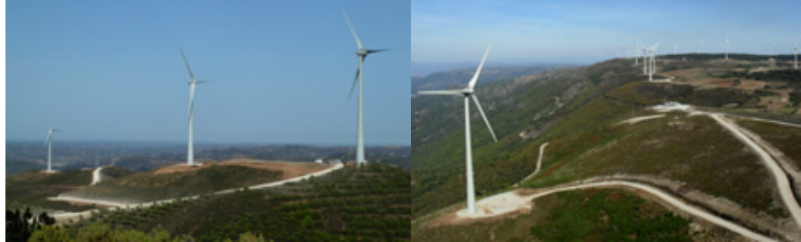
MALHANITO WIND FARM (60 kV connection at the REN Tavira Substation)
